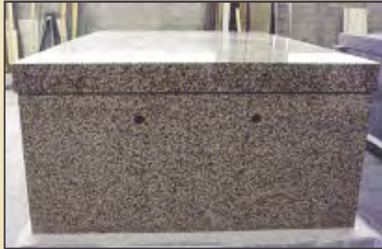
15. The mausoleum is topped with a 6" thick granite roof and two vents are included on the back wall.
