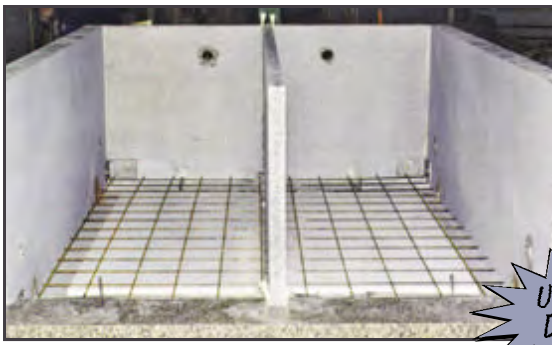
9. The granite divider is placed in the back notch to create two separate crypts.
