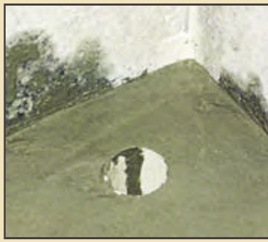
14. The floor is pitched toward drain holes.
