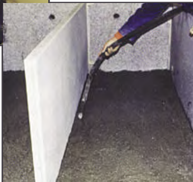
13. The cement floor is smoothed.
